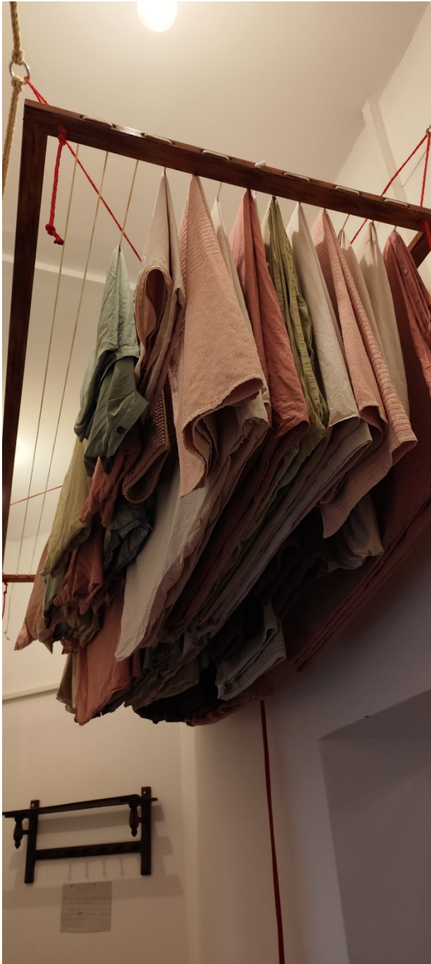
Corridor with ceiling-mounted drying racks
